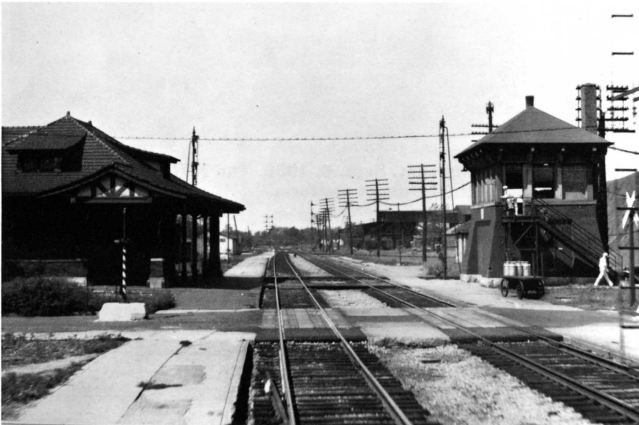
Pana, Ill. looking west along the NYC, Sept. 6, 1936. The C&EI joins in the distance to the right of the tower. The IC crosses at the tower, marked by its home signal semaphores.
